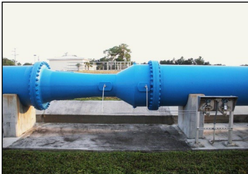
36-inch Venturi Meter (Source: Primary Flow Control)
