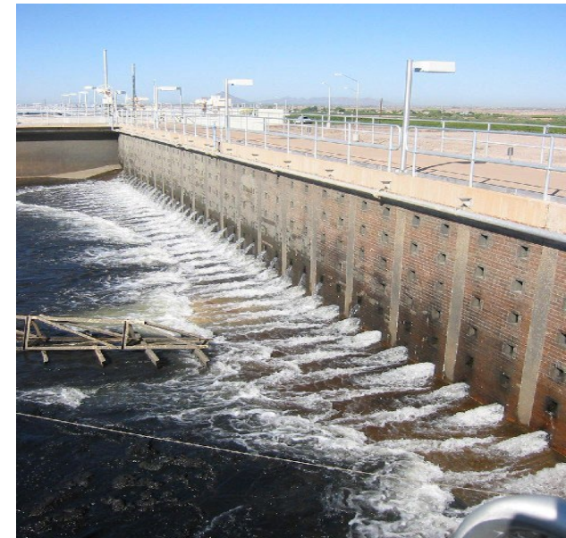
Reservoir or clearwell adjacent to a water treatment plant
